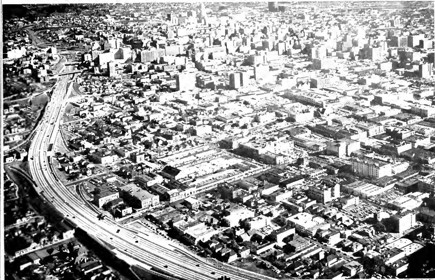
Looking northerly along completed Harbor Freeway from above Las Angeles showing downtown business buildings and Civic Center buildings in center and toward background. The grade separation bridge, foreground left, carries Pico Blvd. under the Harbor Freeway. The four-level traffic interchange structure and Hollywood Freeway are shown background left.
